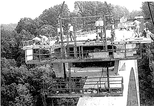
写真-4 Natchez Trace Pkwy Bridge
