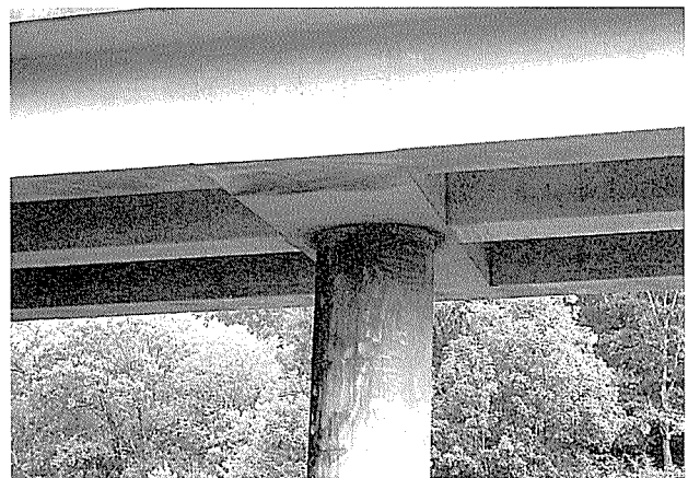
写真-8 South Chicamauga Creek Bridge
