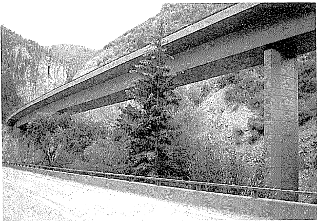
写真-11 Glenwood Canyon Viaduct
