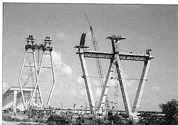
写真-5 Houston Ship Channel Bridge タワー
