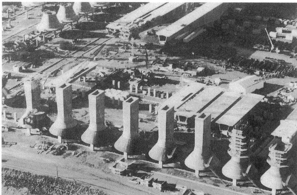
Fig. 18- View of precasting yard with pier shaft units in the forefront
