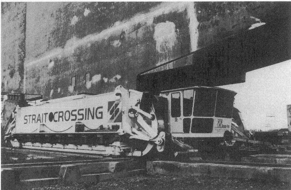
Fig. 12- Huisian Sliding System carrying a main girder unit
