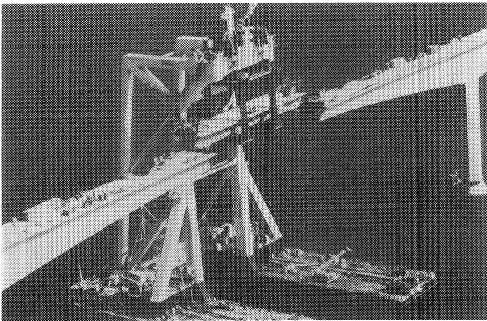
Fig. 16- The Svanen lifting a drop-in unit
