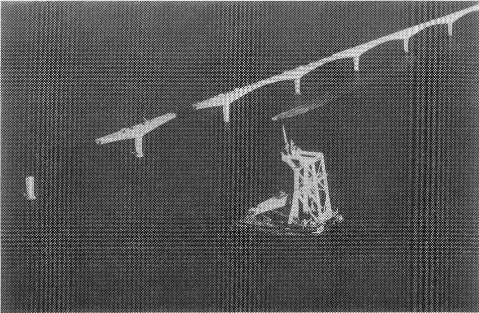
Fig. 15- The Svanen lifting a main girder unit
