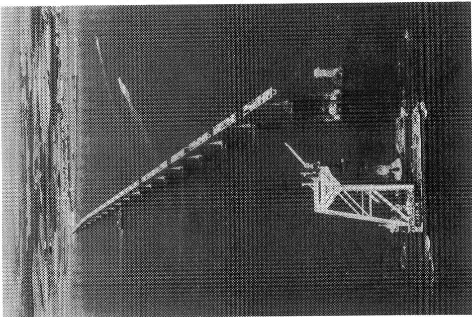
Fig. 13- The Svanen lifting a pier base unit
