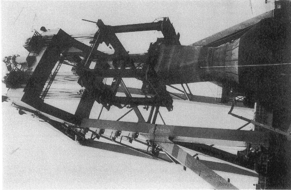
Fig. 14- The Svanen lifting a pier shaft unit
