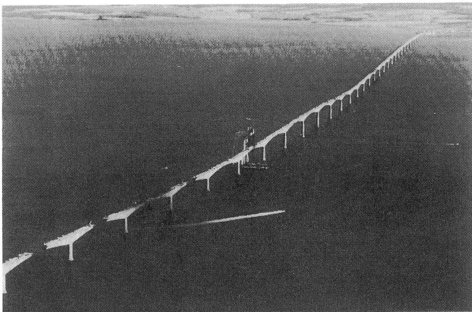
Fig. 22- View of the bridge near the end of marine operations
