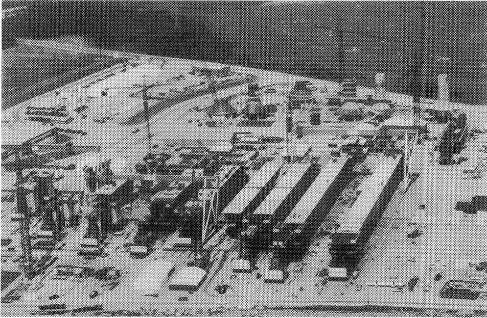
Fig. 19- View of precasting yard with main girder units in the forefront
