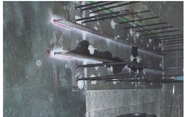
**Fig.3 Epoxy resin grouting**
