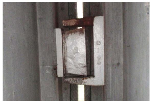
Fig.8 Hinge restrainer
