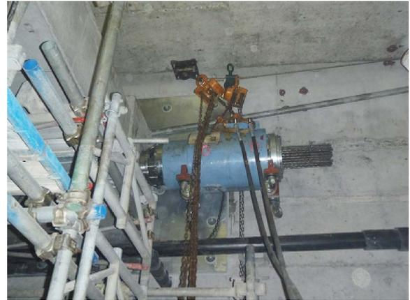
Fig.7 Tensioning work in confined space
