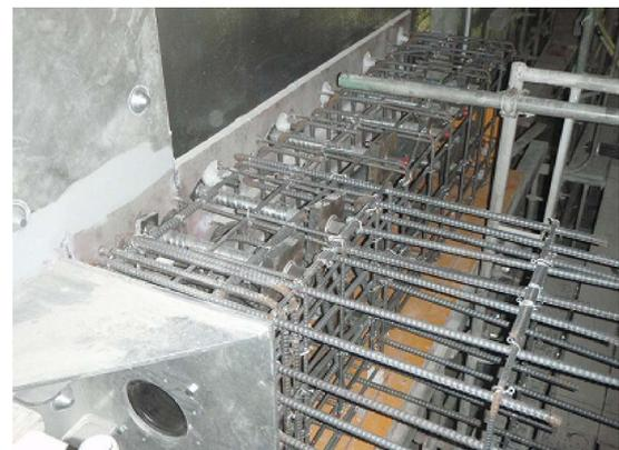
**Fig.4 Reinforcement in anchor block**
