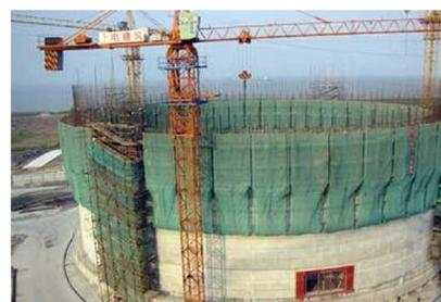
Fig.5 Jumping form method of wall
