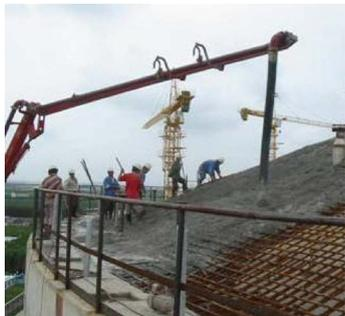
Fig.6 Outer part placing of dome roof
