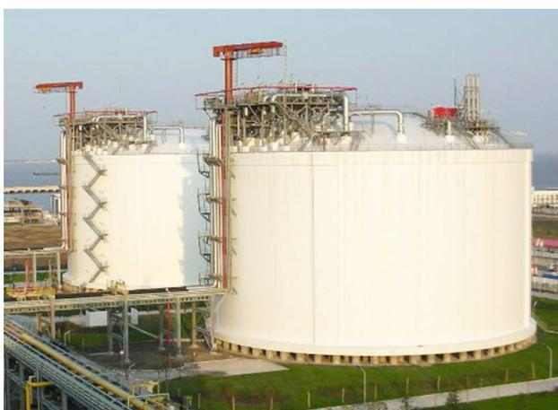
Fig.2 50,000m<sup>3</sup> PCLNG Tanks
