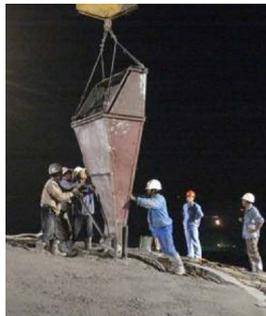
Fig.7 Inner part placing of dome roof
