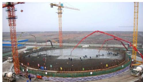
Fig.4 Concrete casting of Base Slab
