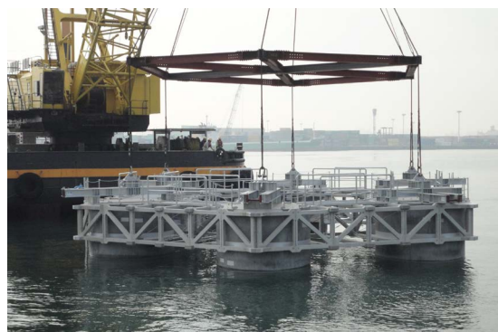
Fig. 8 Lifting of the floating structure
