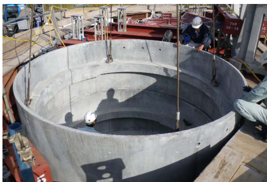
Fig. 6 Construction of the cylinder floating body
