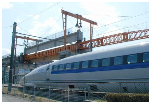
Fig.6 Erection girder method
