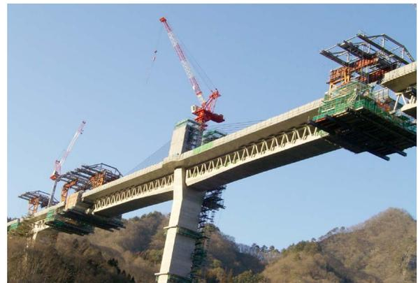
**Fig.8 Balanced cantilever construction**
