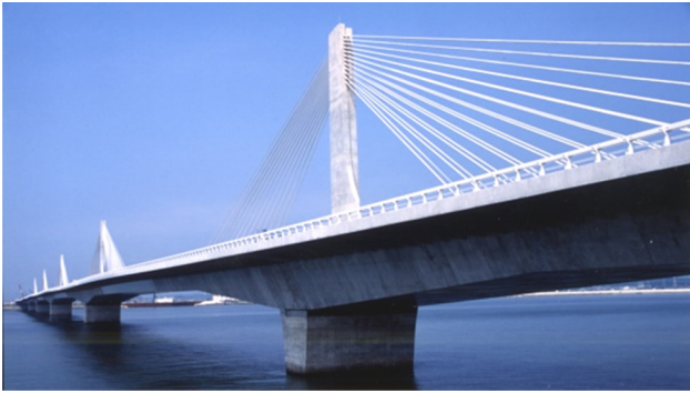
Fig.2 Ibi River Bridge – extradosed bridge with steel-concrete mixed girders
