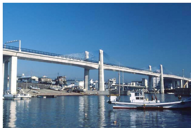
Fig.2 Odawara Blue-way Bridge
