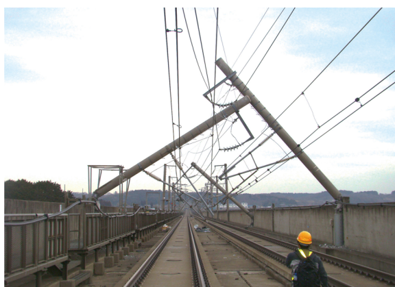
Fig.1 Damage of poles on the viaduct
