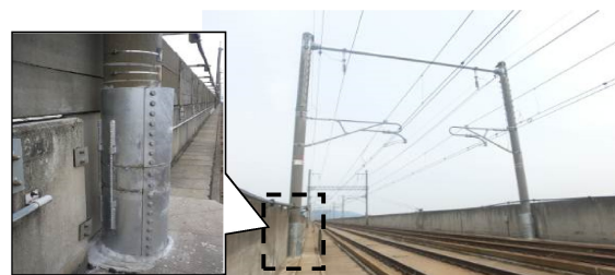
Fig.5 Reinforce pole on the viaduct
