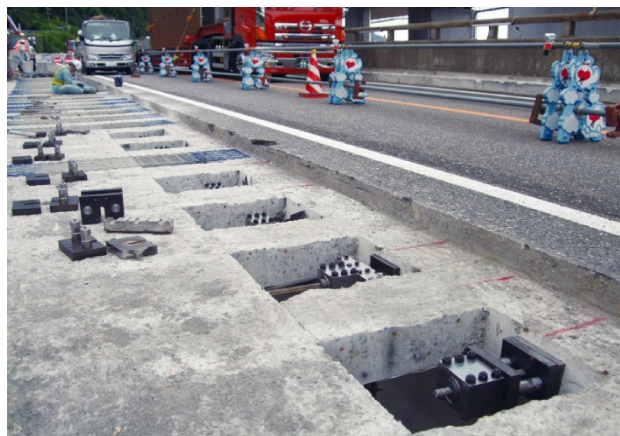
Fig.4 Situation of intermediate fixing
