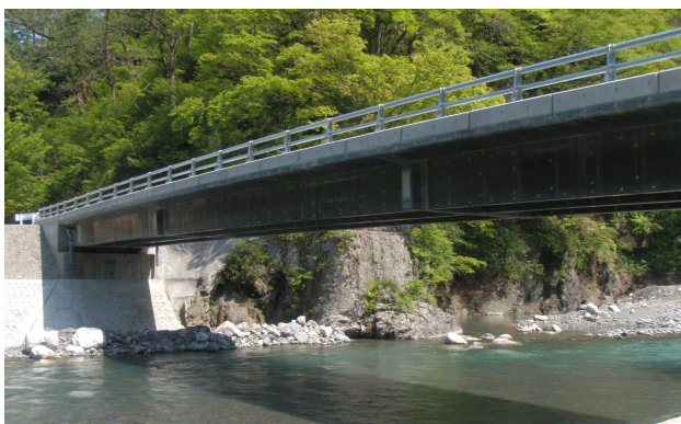
Fig.1 Completed Kotaki River Bridge
