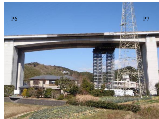
Fig.8 Temporary struts and tendons
