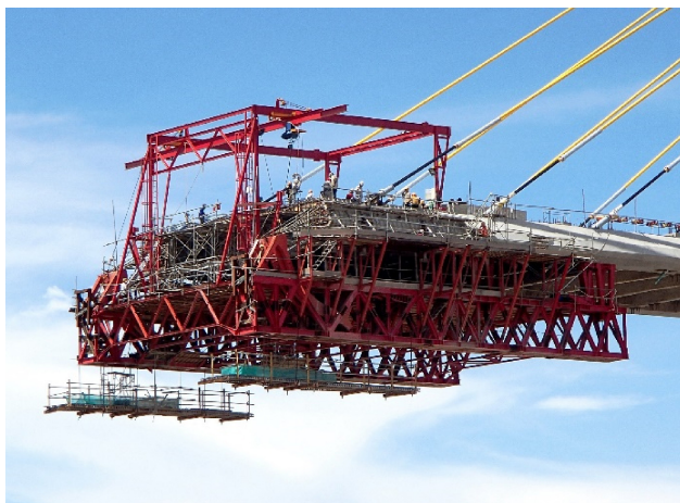
Fig.7 Under-supporting form traveler
