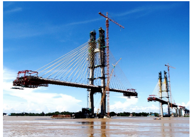
Fig.8 Balanced cantilever erection
