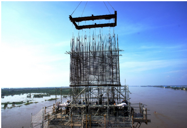
Fig.10 Prefabricated rebar cage
