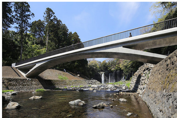
Fig.1 Takimi Bridge (flat balanced arch structure)
