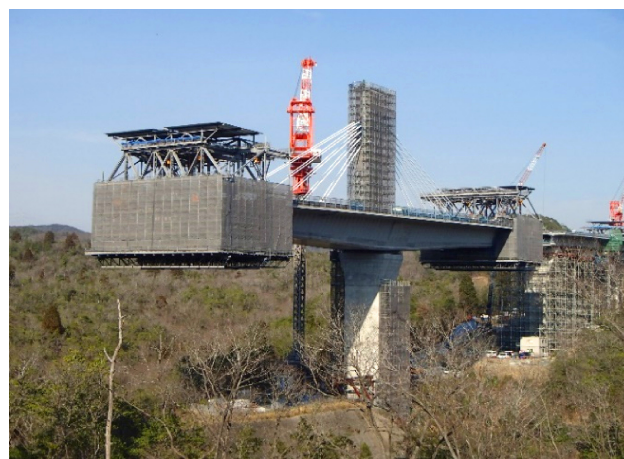
Fig.10 Cantilever erection by extra-large traveler
