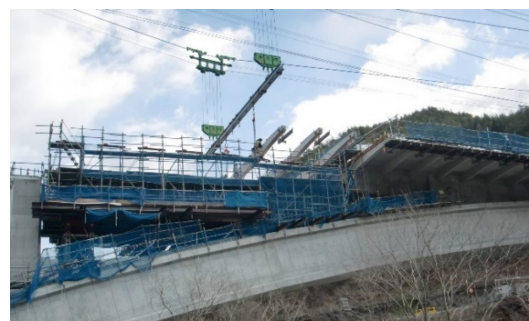
Fig.7 Installing the horizontal ribs
