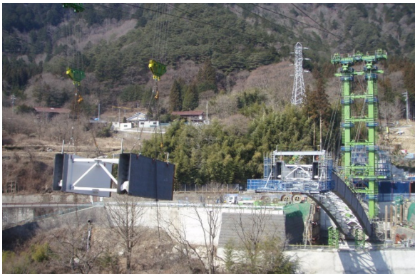
Fig.5 Erection of steel member
