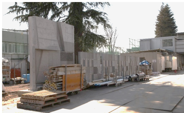
Photo 4. Mock-ups at the construction site
