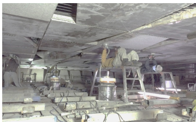
Photo 5. On-site process of finishing the concrete ceiling surface. This situation resembled that of Michelangelo's fresco ceilings at the Sistine Chapel
