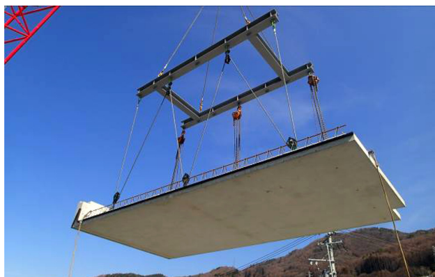
Fig.11 Fitting used to hoist PCa floor member
