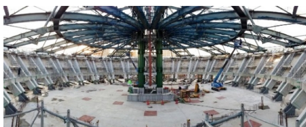
Fig.10 After uplifting (completion after 8 hrs of uplifting)
