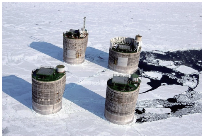
Figure 4 Concrete platform in ice, Sakhalin II (Reference 3)
