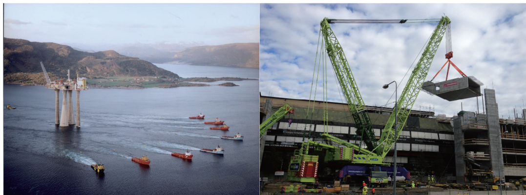
Figure 2 The Troll A Platform being towed out of a Norwegian fiord, displacing 1,000,000 t, and lifting 250 t on shore
