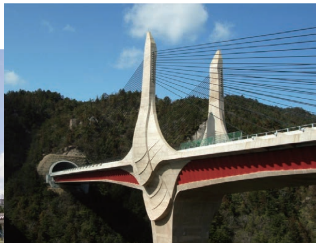
Ohmi-Ohdori Bridge on the New Meishin Expressway
