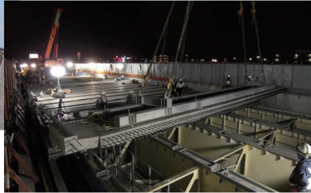
Mukaizano Bridge (Kyusyu Expressway) Concrete Slab Replacement in Heavy Traffic Expressway
