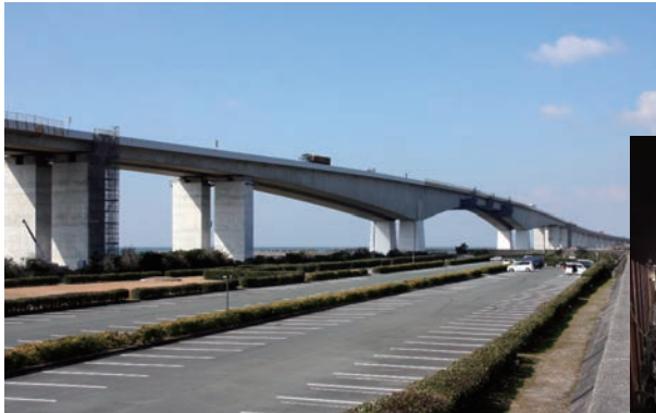
Hamana Bridge (National Route 1) Seismic Retrofit for Rigid-frame Bridge with Central Hinge
