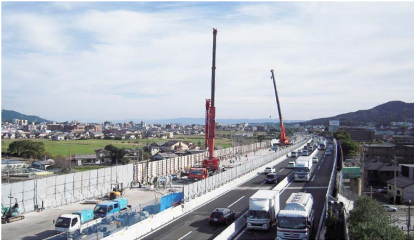
Fig.4 Slab replacement under traffic restriction
