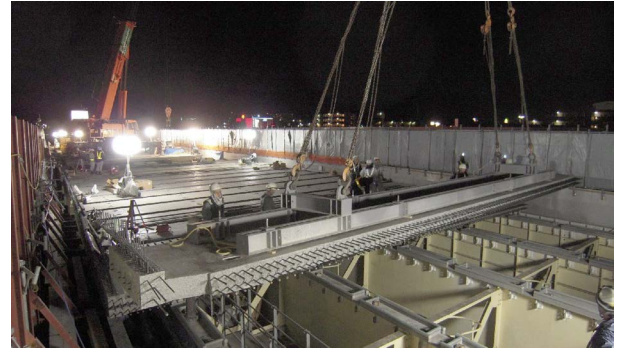
Fig.5 Erection of PCa slab panels
