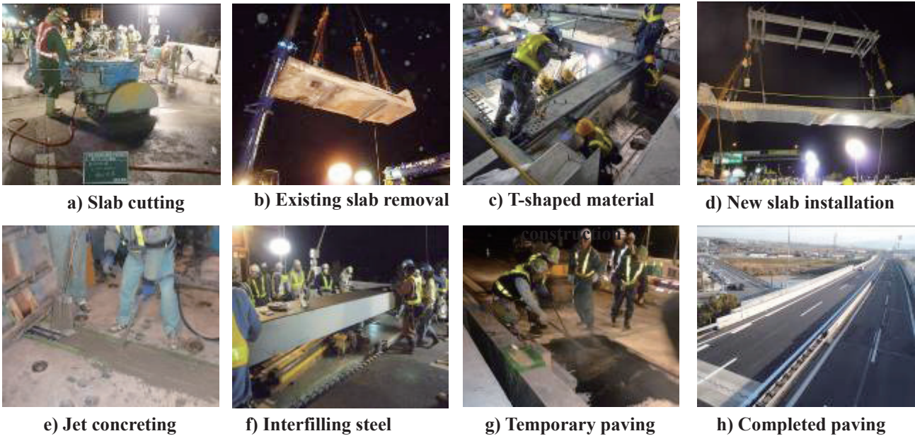
Fig.6 Stages of intensive construction work at second term
