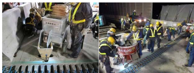
Grouting of precast slab to girder
