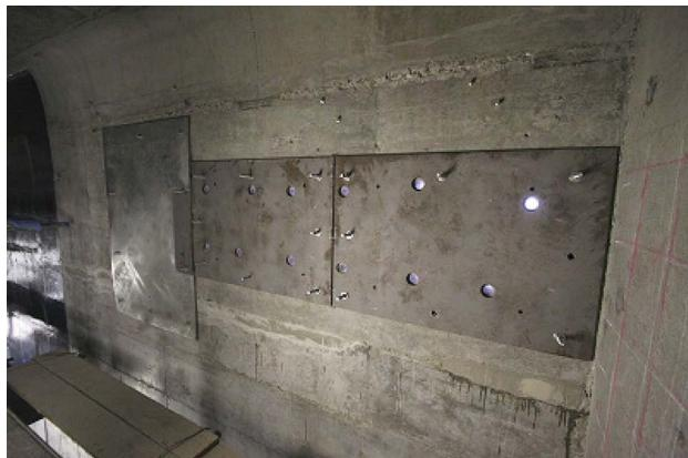
**Fig.2 Locations of drilled holes in girder web**
