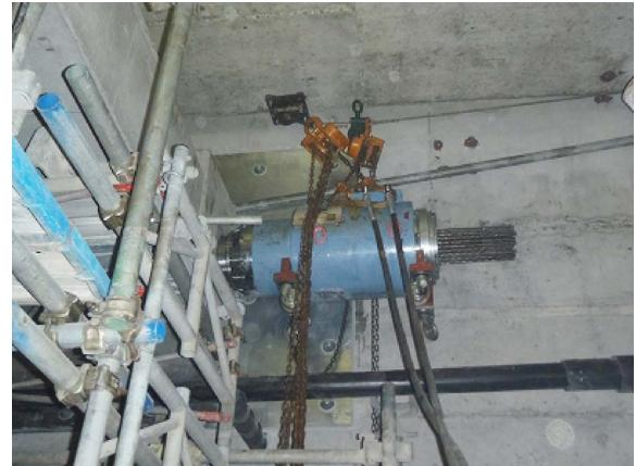
**Fig.7** Tensioning work in confined space
