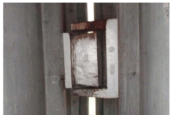
**Fig.8** Hinge restrainer
