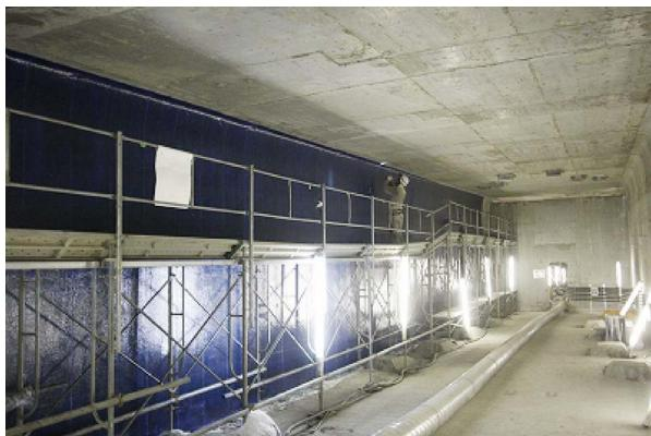
**Fig.9 Carbon fiber sheet reinforcement inside box girder**
