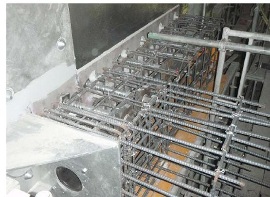
**Fig.4 Reinforcement in anchor block**
