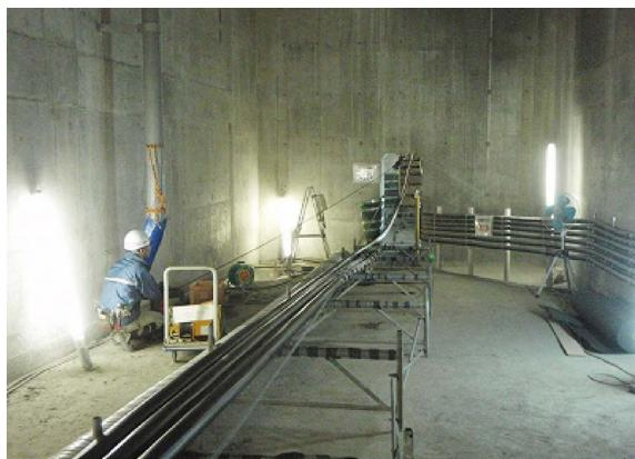
**Fig.6** Insertion of external tendons into box girder
