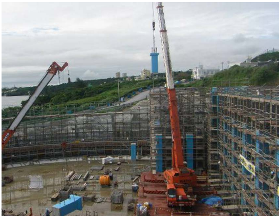
Fig.12 PCa pillar work
