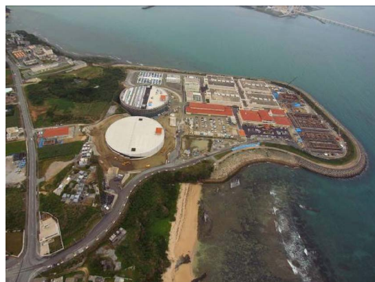
Fig.1 The Shin-Ishikawa Water Treatment Plant
