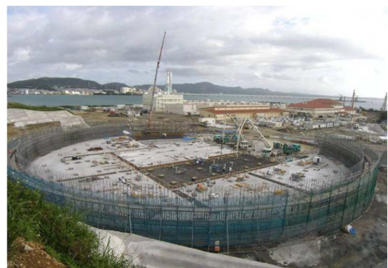
Fig.6 Base slab work
