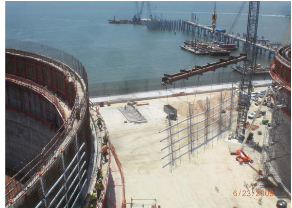
Fig. 7 Installation of prefabricated rebar and sheath
