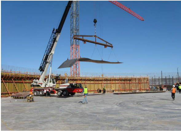
Fig. 4 Installation of base plate
