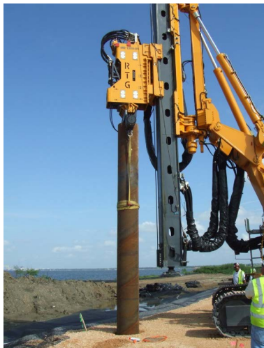
Fig. 2 Driving piles by vibratory hammer
