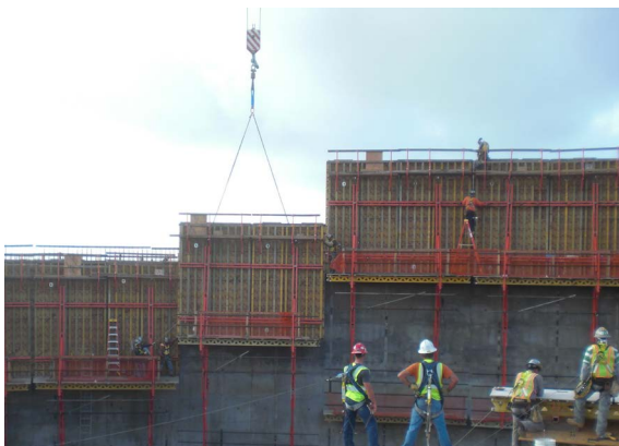
Fig. 6 Jumping-up of climbing form
