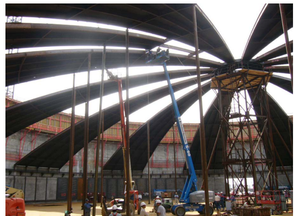
Fig. 9 Installation of roof block
