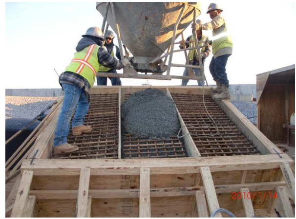
Fig. 12 Full-scale test for decision of slump
