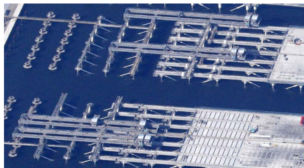
Fig. 14 Construction of PC girder-slab structure
