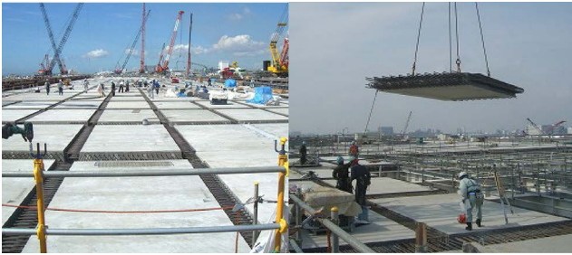
Fig. 6 Installation of PCa slabs
