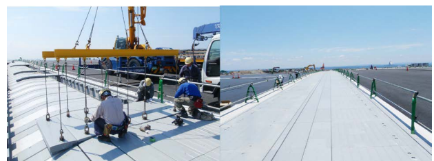
Fig. 11 Installation of expansion joint
