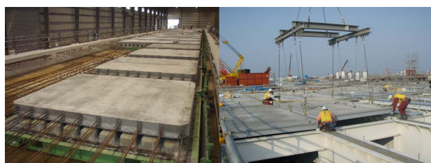
Fig. 8 Construction of UFC slabs
