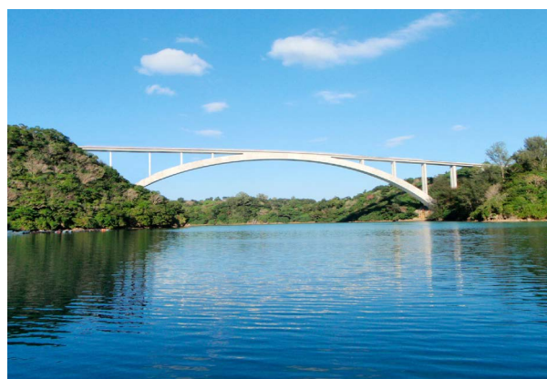
Fig.10 Side view of the Warumi-Ohashi Bridge
