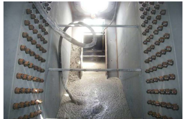
Fig.6 Filling concrete into steel box arch
