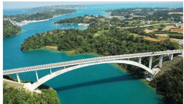
Fig.1 The Warumi-Ohashi Bridge
