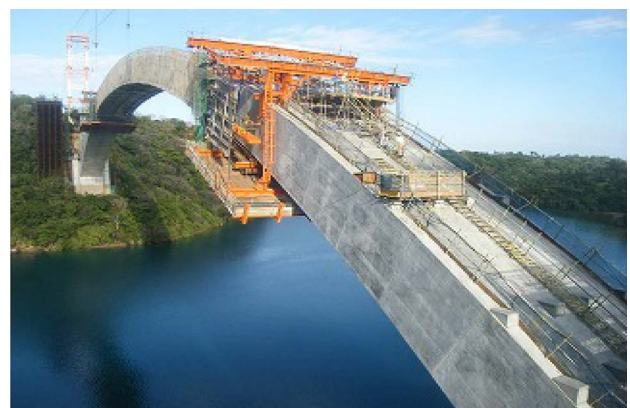
Fig.7 Concrete lapping of composite arch
