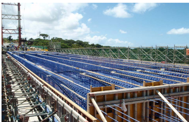
Fig.8 Installation of tendon and rebar
