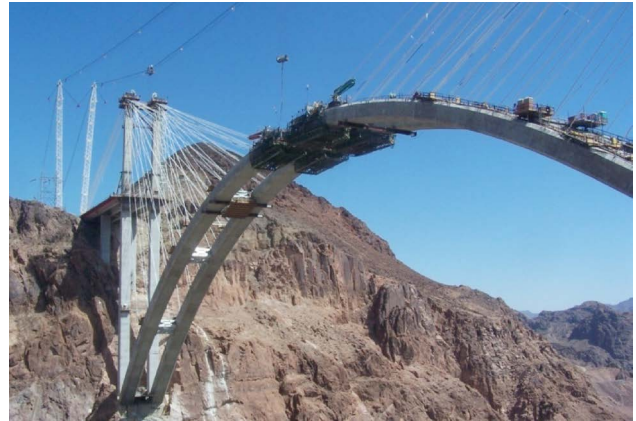
Fig.6 Arch rib cantilever construction
