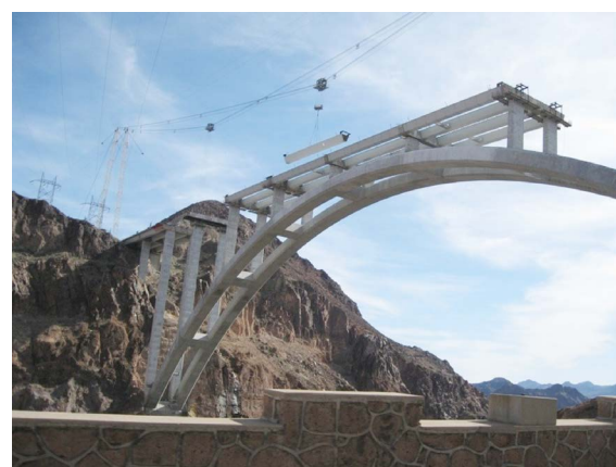
Fig.9 Tub Girder erection
