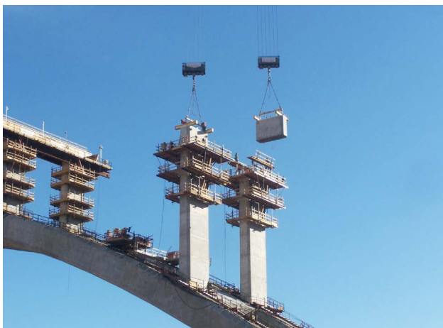
Fig.5 Pier column segment erection
