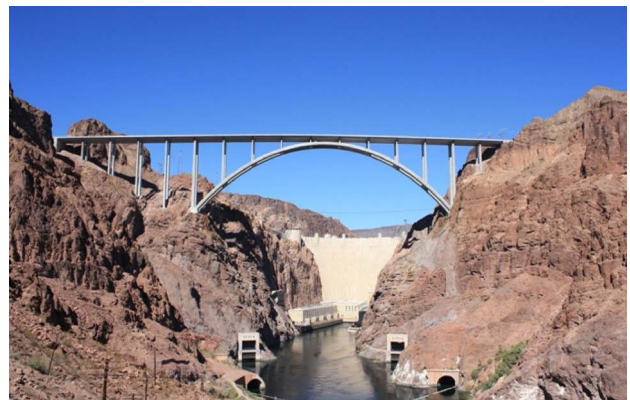
Fig.1 Hoover Dam Bypass Colorado River Bridge
