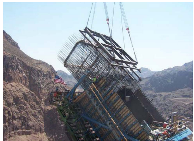
Fig.7 Arch rebar cage
