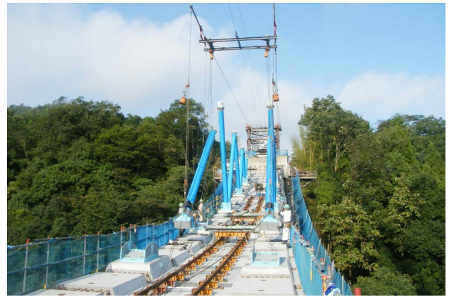
Fig.7 Erection of steel diagonal members
