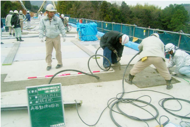
Fig.9 Concrete compaction by revibrating
