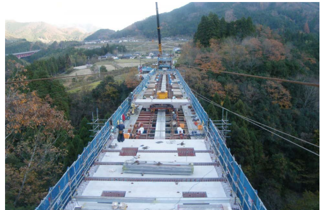
Fig.8 Erection of the upper girder deck
