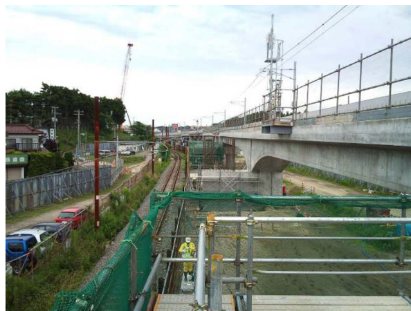
Fig. 7 Construction situation (Phase 2)
