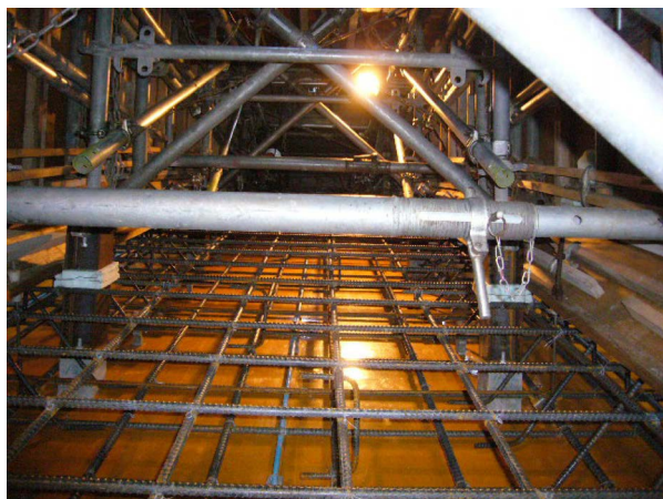
Fig. 6 Formwork in box girder
