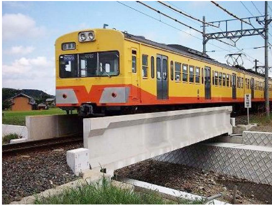
Fig. 1 Kayogawa UFC railway bridge
