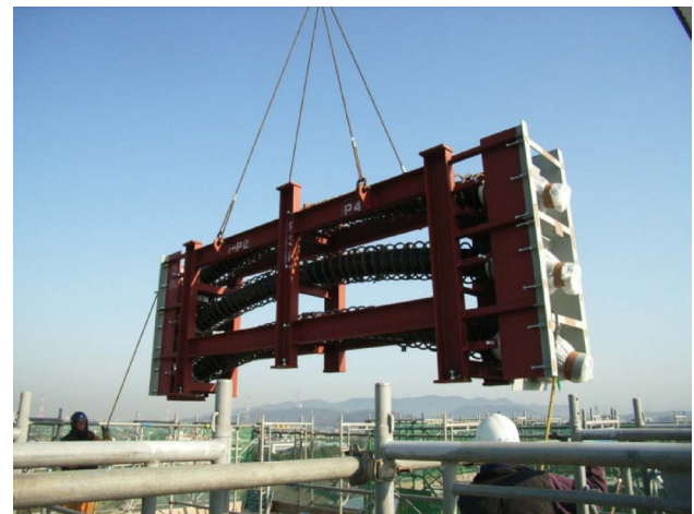
Fig.4 Prefabricated saddle of stay cables
