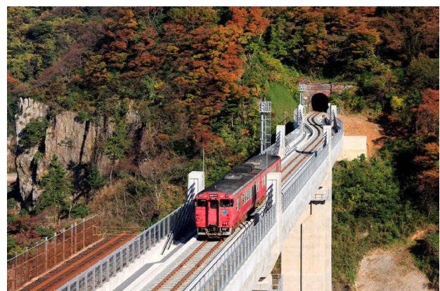
Fig.11 New Amarube Bridge (2010-)
