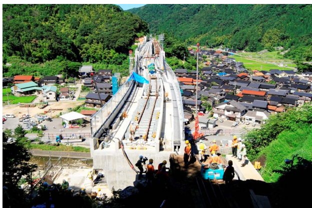
Fig.9 After sliding of girder
