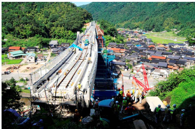
Fig.8 Before sliding of girder
