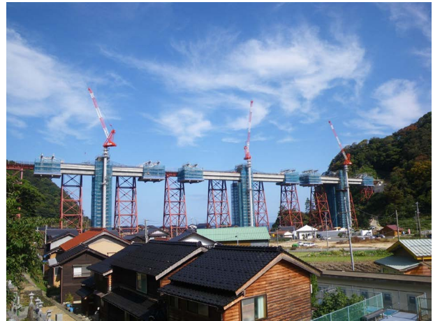
Fig.6 Cantilever construction at P1 to P3
