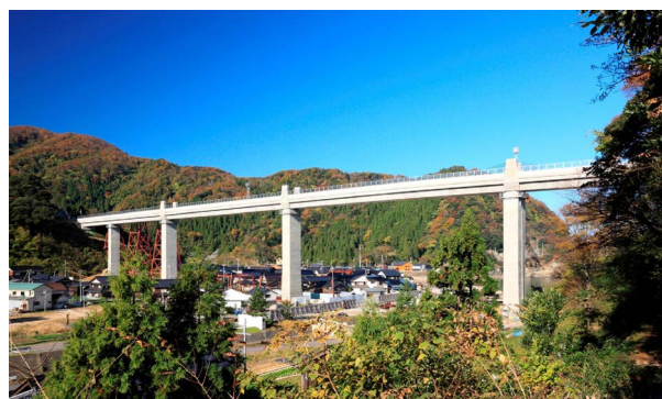
Fig.1 New Amarube Bridge (2010-)
