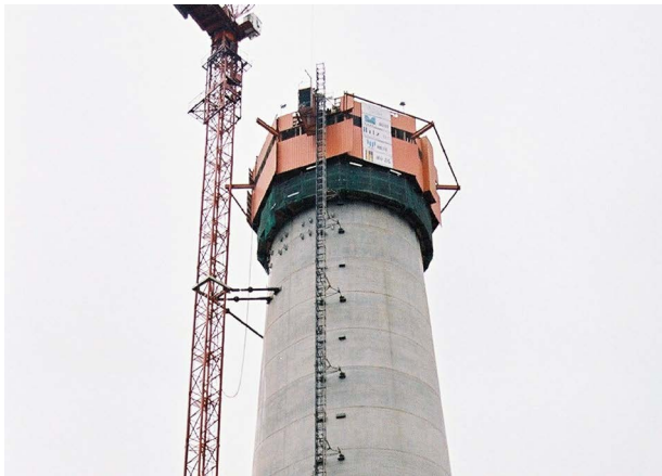
Fig. 3 Self-climbing form system for Tower
