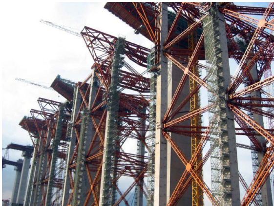
Fig. 7 Concrete Side span Falsework
