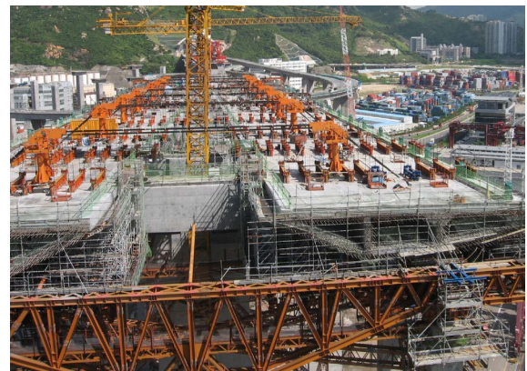
Fig. 8 Falsework of concrete deck
