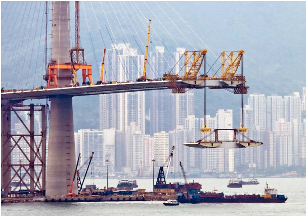
Fig. 10 Erection of main span segment
