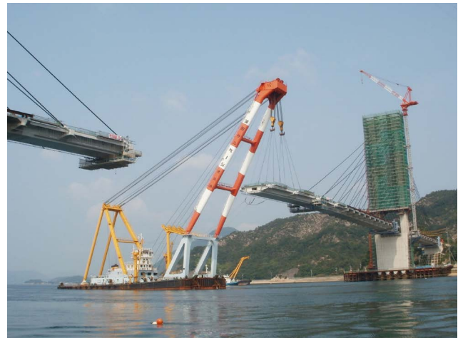
Fig.8 Cantilever erection (steel girder)
