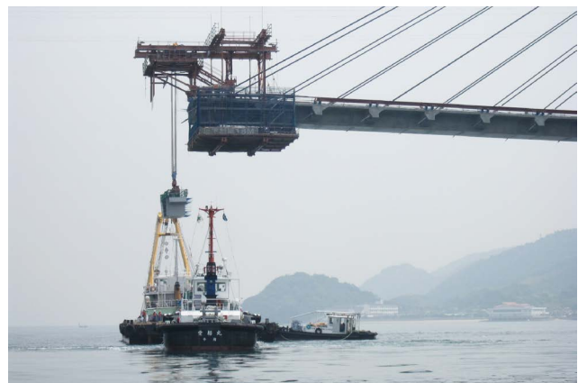
Fig.7 Connection girder Erection
