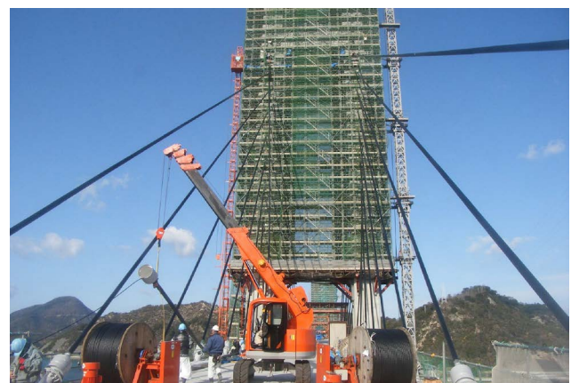
Fig.9 Stay cable construction
