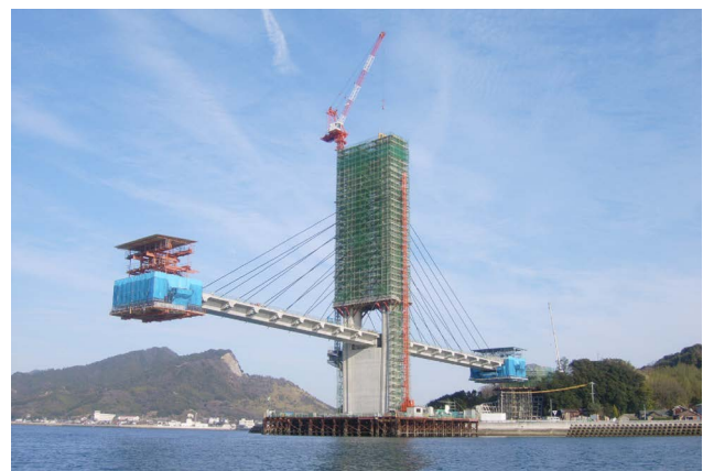
Fig.5 Cantilever erection (concrete girder) onstruction at P2
