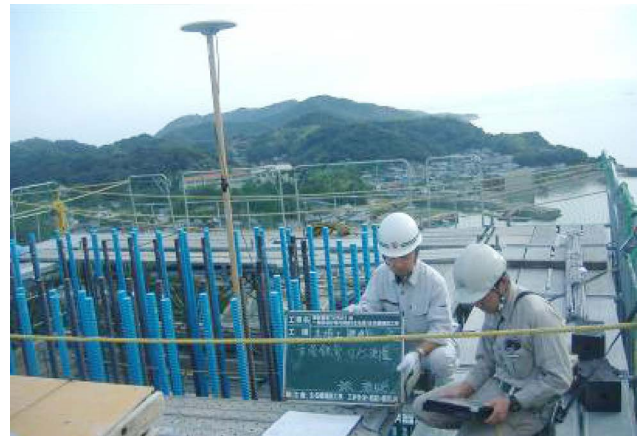
Fig.4 Quality control using GPS method
