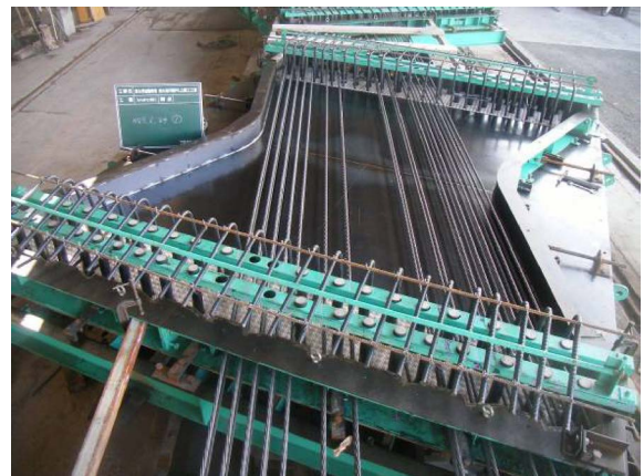
Fig.7 Prefabrication stage of the panel
