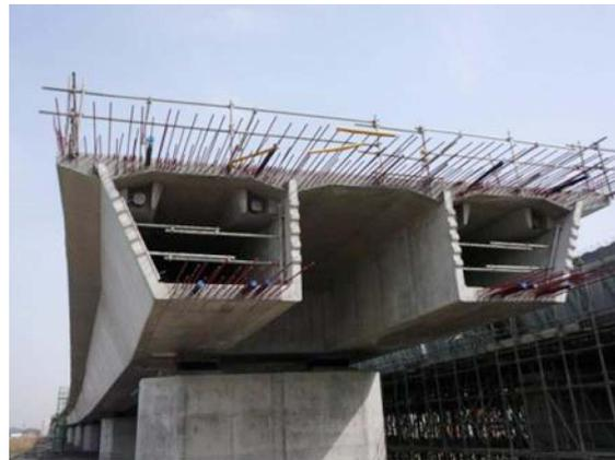
Fig. 13 Cross section
