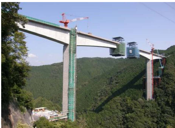
Fig. 6 Balanced cantilevering using ultra-large travelers
