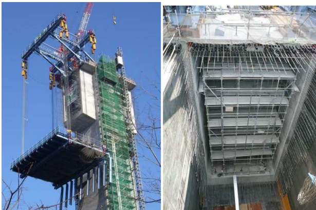
Fig. 5 Ultra-large traveler: Assembly and Internal falsework
