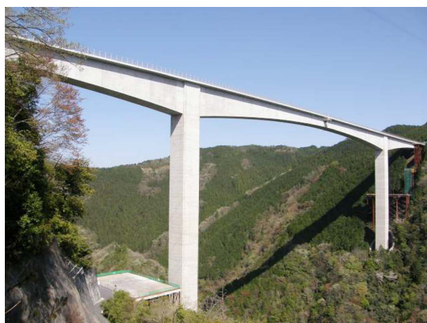
Fig. 7 Shintabisoko Bridge (after completion)
