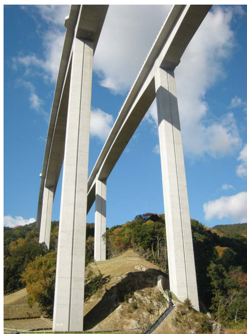
Fig.8 Sanagawa Bridge (upward view)
