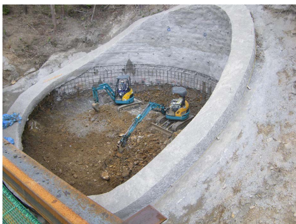
Fig.7 Structural excavation like cutting a bamboo
