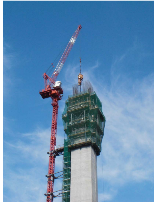
Fig.5 Construction of bridge pier (Use of climbing form and concrete placement with buckets)
