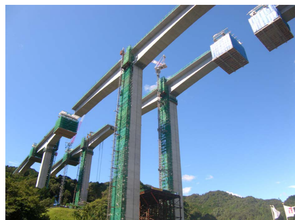
Fig.6 Construction of superstructure
