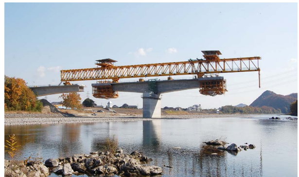
Fig. 3 Construction by the P&Z method
