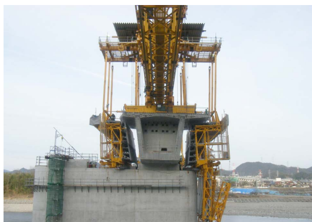
Fig. 9 Single-door form opened to clear the pier
