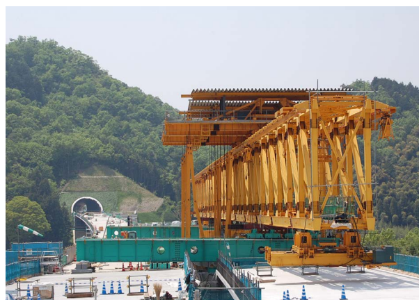
Fig. 8 Launching gantry shifted from left to right
