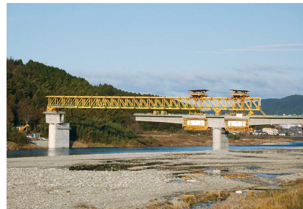
Fig. 7 Launching gantry in transfer
