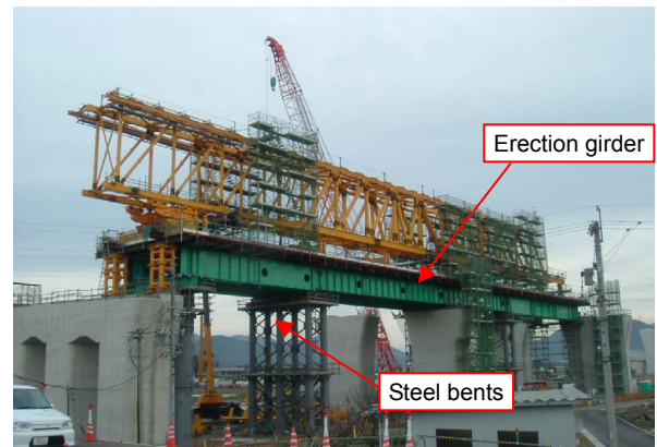
Fig. 6 Launching gantry assembly
