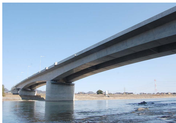
Fig. 10 Completion of the bridge
