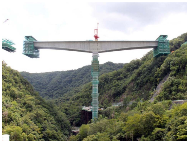
Fig. 5 Cantilever erection
