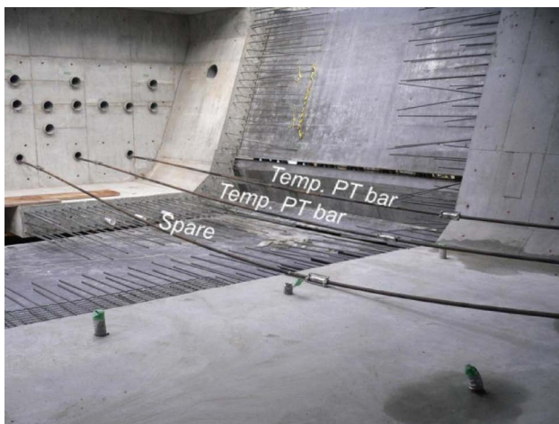
Fig. 8 Temporary PT bars (before tensioning)
