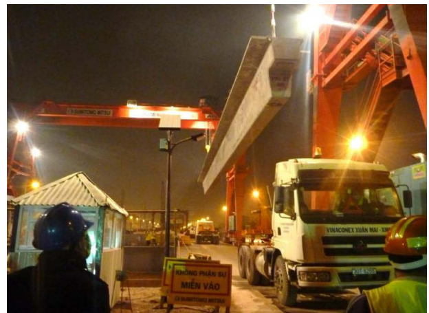
Fig.10 Erection of super-t girder
