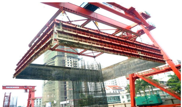
Fig.5 Form of pile cap
