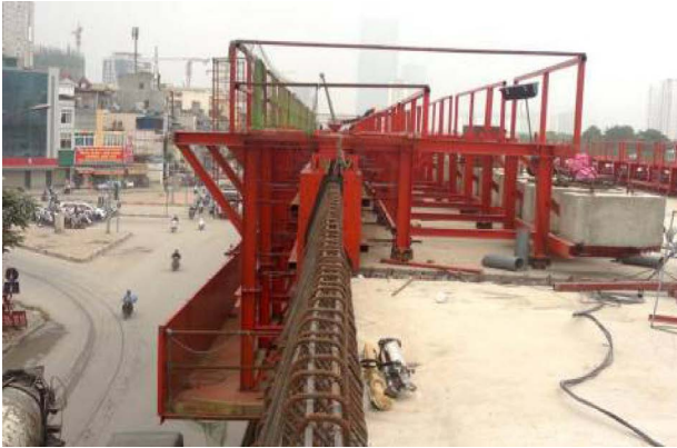
Fig.12 Parapet work by gondola
