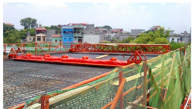
Fig.11 Finishing of slab-surface concrete
