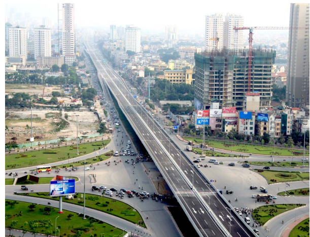
Fig.13 Completion and traffic open
