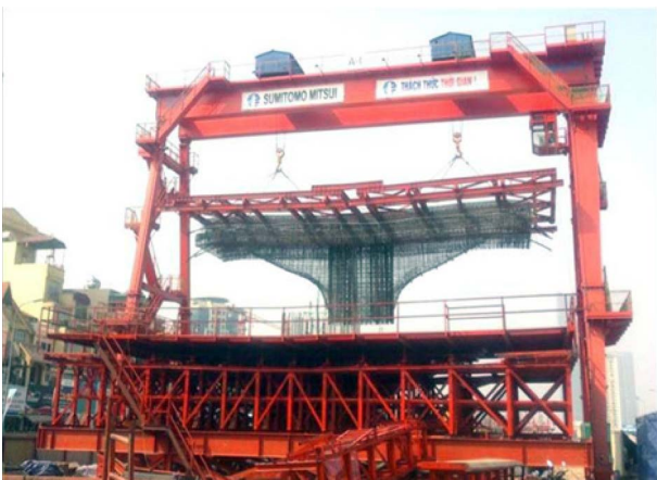
Fig.8 Installation of pre-assembled rebar
