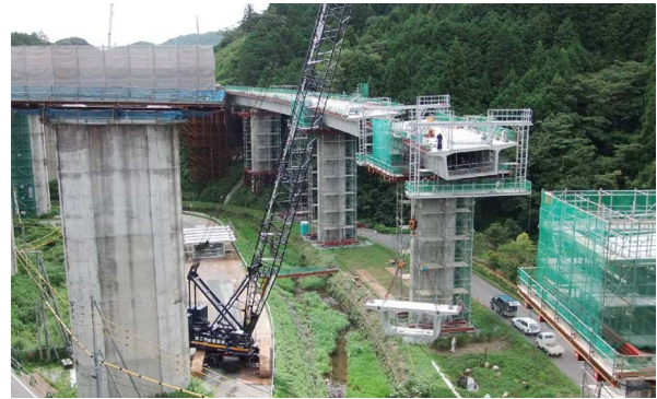
Fig.7 Cantilever erection using a crawler crane
