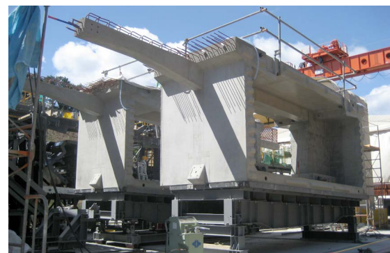
Fig.8 Short line match casting method
