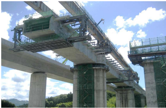
Fig.5 Cantilever erection using erection girder
