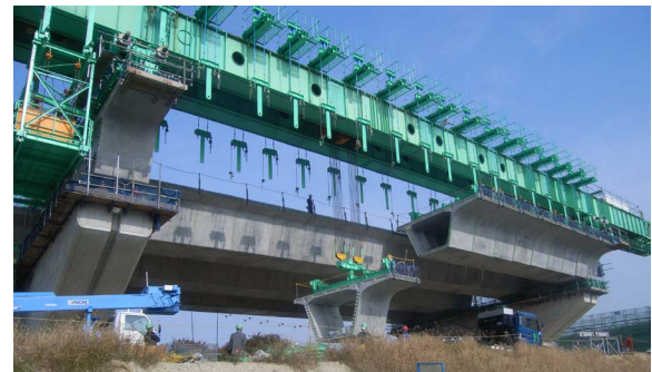
Fig.2 Span-by-span erection using hangers
