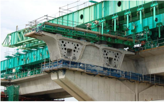
Fig.4 Connecting pier head segments first with transverse girders
