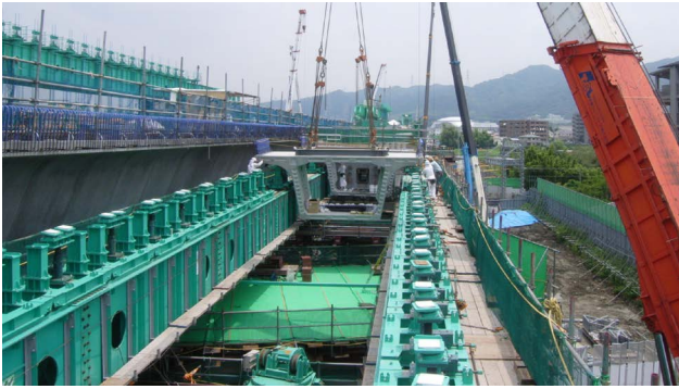
Fig.6 Span-by-span erection using supports
