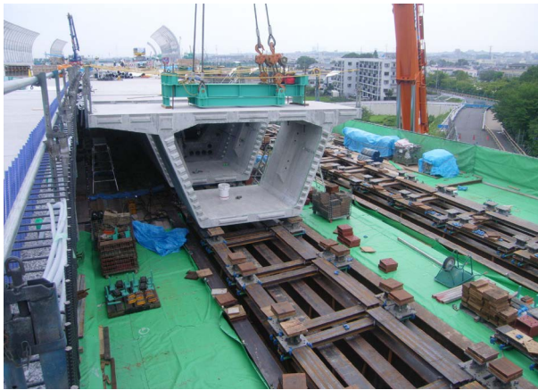
Fig.7 Erection using staging
