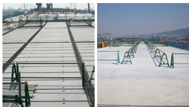
Fig. 11 Precast panels Fig. 12 Cast-in-situ slab
