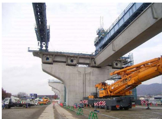
Fig. 10 Transversal movement of the girder
