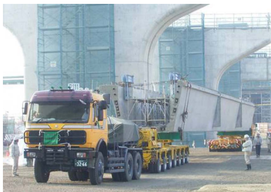
Fig. 8 Transportation of the U-girder
