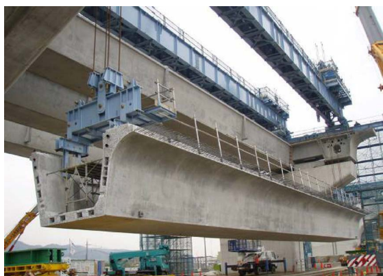
Fig. 9 Erection of the U-girder
