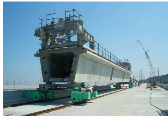
Fig. 7 Transportation of the girder
