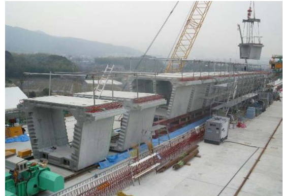
Fig. 6 Assembling the segments
