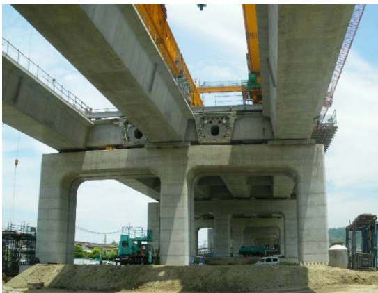
Fig. 9 Transversal movement of the girder
