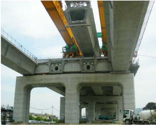
Fig. 8 Erection of the girder
