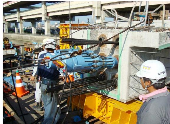
Fig. 8 Cable tensioning
